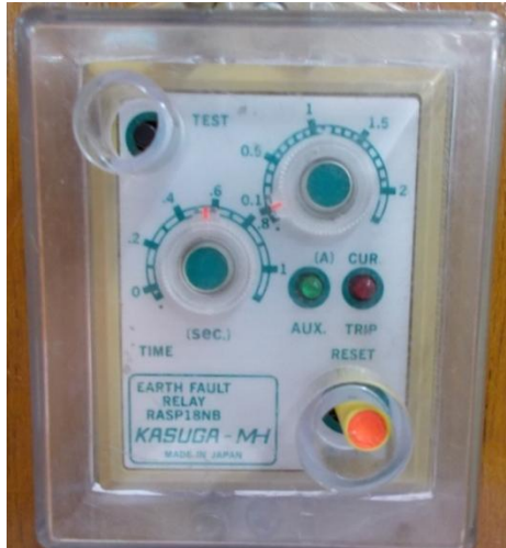
Gambar Earth Fault Relay
