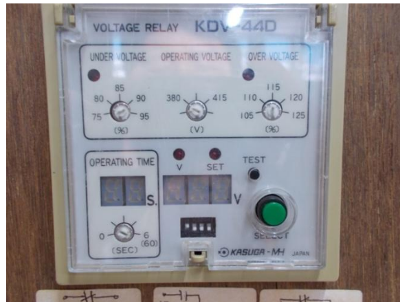
Gambar Voltage Relay Kasuga MI 1 KDV 44D
